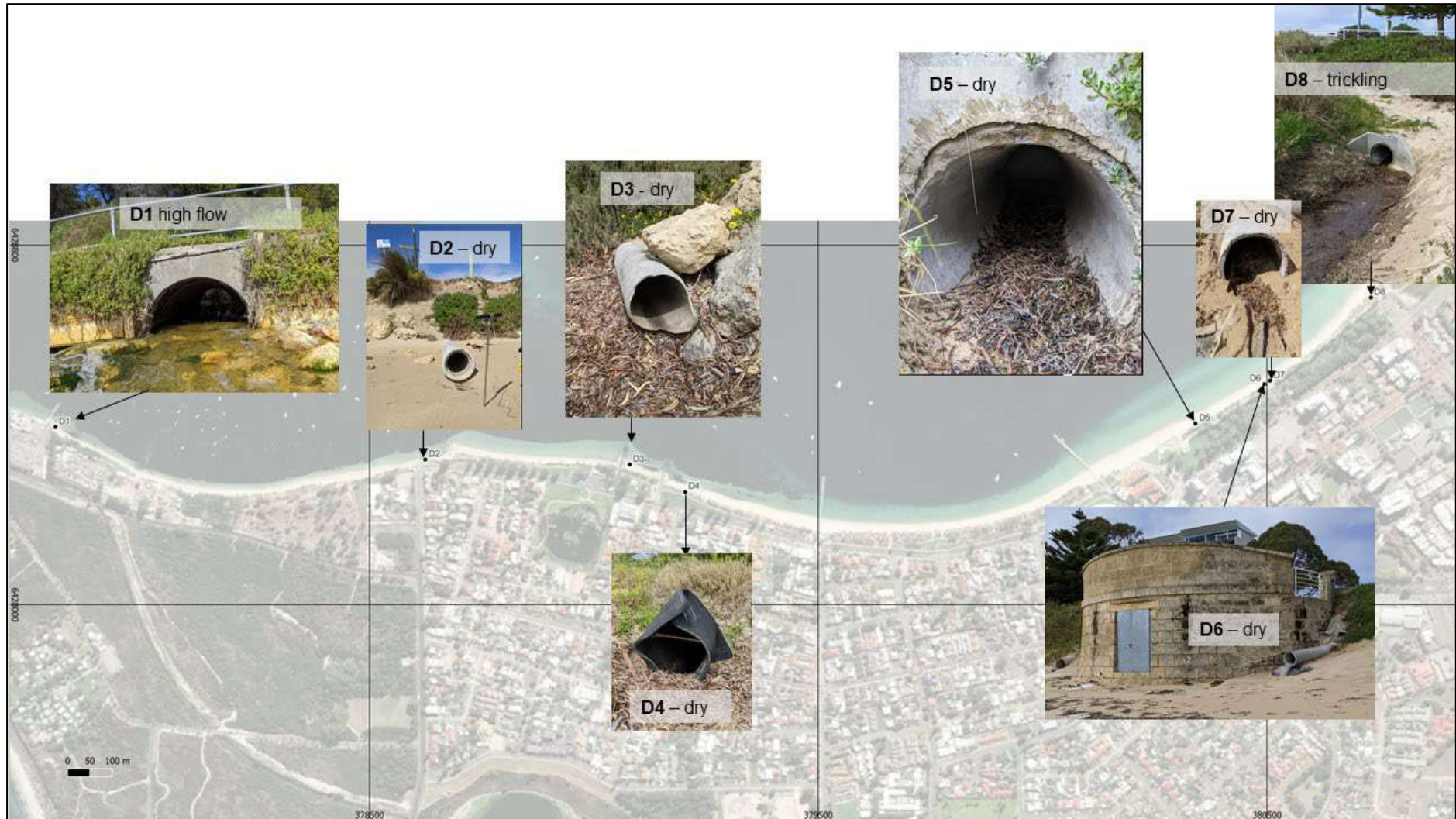
Figure 5. Stormwater drains D1 through D8 re-visited on 14 September 2022. Compare with Figure 3, which was during wetter conditions.
