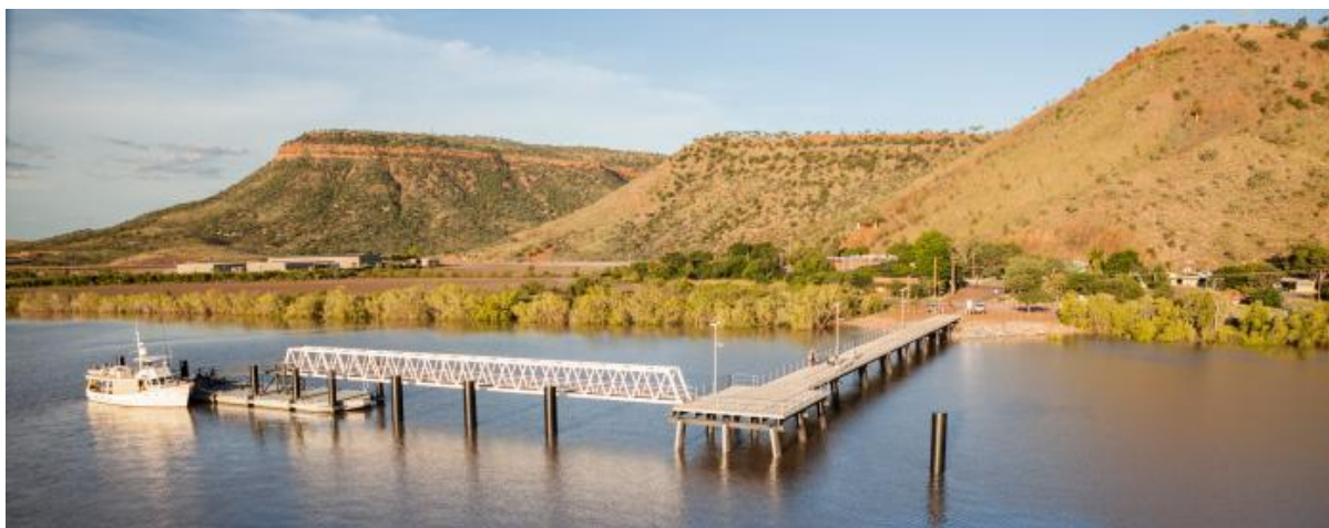
Figure 5. Anthon's Landing in Wyndham, Kimberley. Source Maritime Constructions, photo by David Wilcock Photography.
